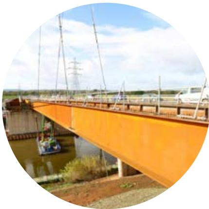
The size of the crane enabled the final pairs of girders to be lifted over the river at a radius of 82m from the crane. To eliminate the risk of the crane boom collapsing onto power lines, it was also moved to a new position part way through the installation.
