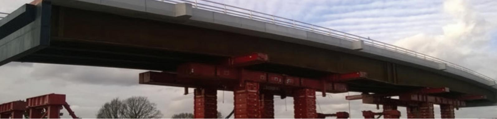
**The Thorley Lane replacement bridge, crossing the M56 was assembled in an area approximately 200m from its final position and adjacent to the live carriageway.**
