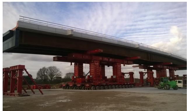
The completed bridge being jacked clear of the temporary supports.
