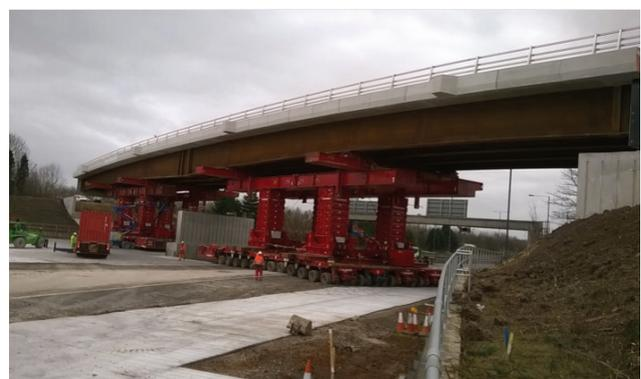
Lowered into its final position, SPMTs removed and the M56 reopened
