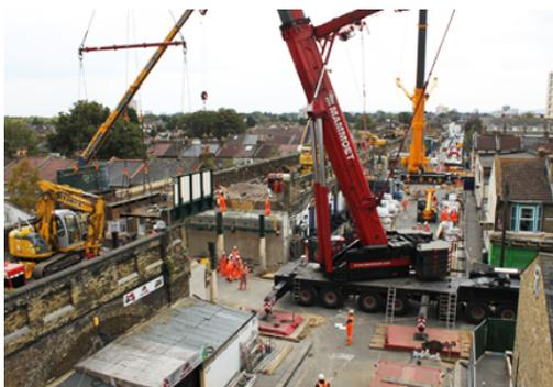
The existing bridge decks were removed in three sections, using the crane to remove one part at a time. The replacement bridge was fabricated and delivered in two sections; these were lifted into position such that the holding-down bolts for the bearings aligned with pre-formed sockets in the bearing plinths.
