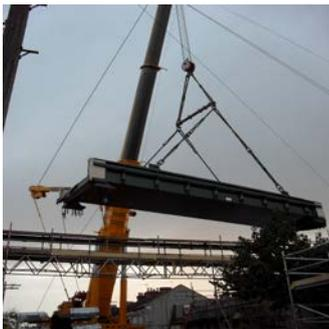
The project involved the replacement of four bridges on the Gospel Oak to Barking railway line over three weekends, during 50hr possessions of the railway. The project is part of a wider scheme by Network Rail to ensure railway infrastructure is upgraded to suit current traffic loadings. The Gospel Oak to Barking line is heavily used by freight as well as passenger trains, so it was deemed appropriate to replace the 120 year old bridges.
