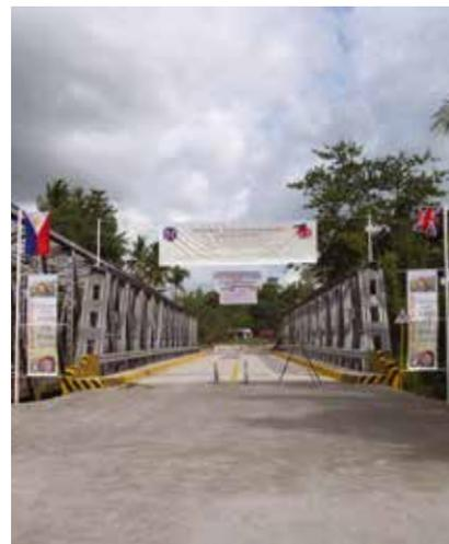
Truss bridges can be single or double lane, according to requirements, and are fully galvanised for protection against the elements. Walkways can be created within the trusses, using handrails to separate pedestrians and traffic. Alternatively, walkways can be fitted outside the trusses for greater safety, allowing the deck between the trusses to be used entirely for traffic.
